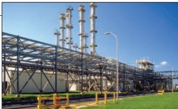
FIGURE 2. CH2M Hill is providing EPC services at the Mitsubishi polysilicon plant in Alabama
