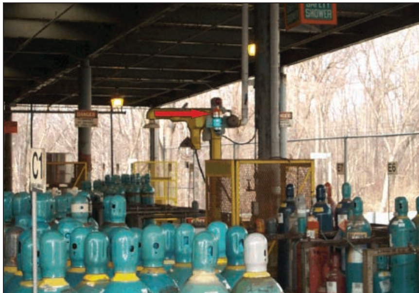
FIGURE 3. LED-based location lighting is useful for signaling the location of safety showers and eyewashes, since they remain visible in daylight conditions
